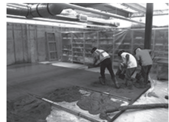
Contractors pour cement for new compact storage to house archeological collections.
