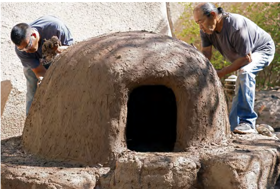
Warren and Robert Edaakie working together to repair the Maxwell horno (photograph by Toni Gentilli)
