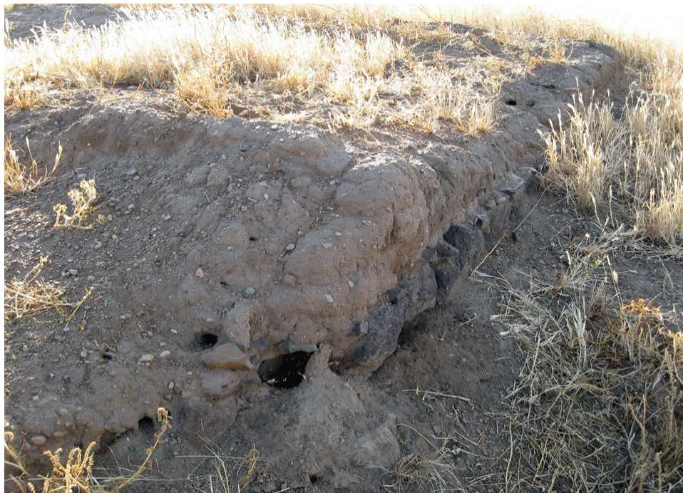
Figure 6.9. Palacios Site, 2012: exposed adobe wall showing cimientos . The latter can be seen in the right half of the photograph.
