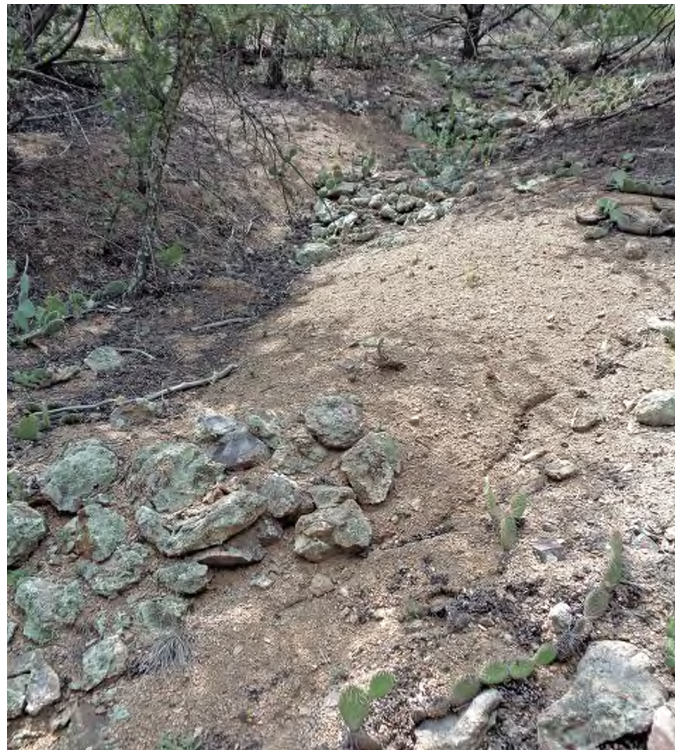
Figure 22. CCC-built check dams in the Juan Tabó watershed.
